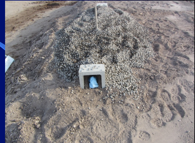
Excavation backfilled and topped with pea gravel
